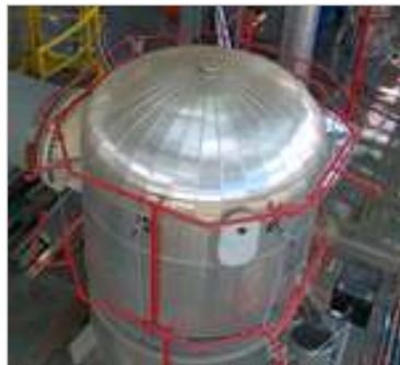
On High Fire Hazards
